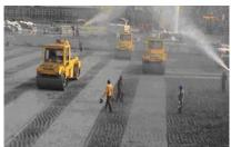
Fig. 15: Curing RCC
