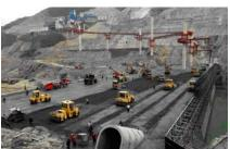
Fig. 14: Spreading and compaction of RCC
