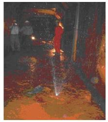
Fig. 19: Water leaking in the dam corridor
