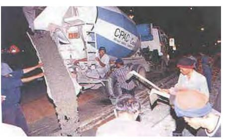
Fig. 6 Pavement Repair with High Early Strength Concrete
