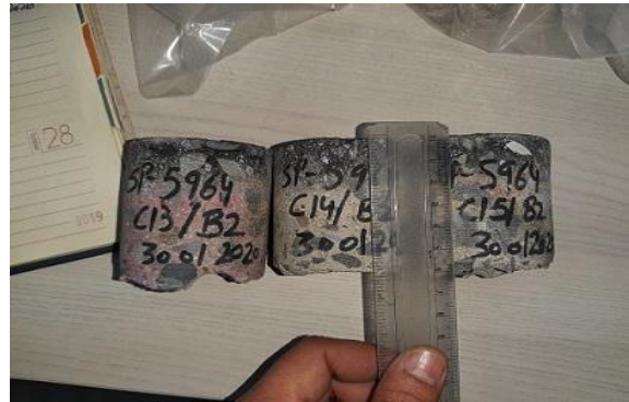
Fig. 5 – Colour change to a blackish grey colour in the cover region of concrete bearing pedestal B2.
