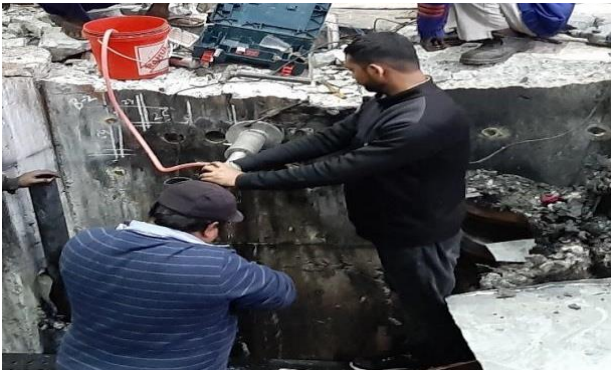
Fig. 4 – Extraction of cores from the concrete bearing pedestal B-2
