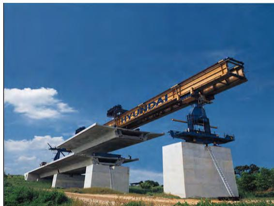
Fig. 4 Installation of 25m long precast prestressed box girder
