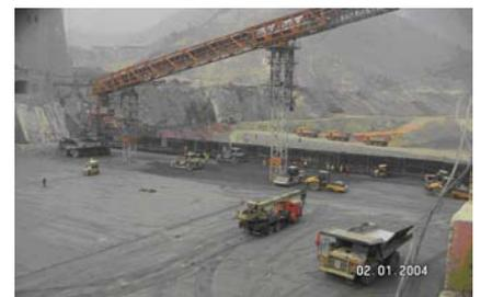
Fig. 13: Belt conveyor and transportation system vehicles
