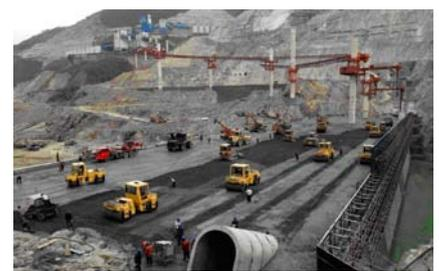
Fig. 14: Spreading and compaction of RCC
