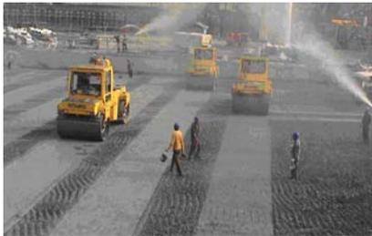
Fig. 15: Curing RCC
