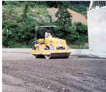
Fig. 3 Roll Compacted Concrete with the Compaction
