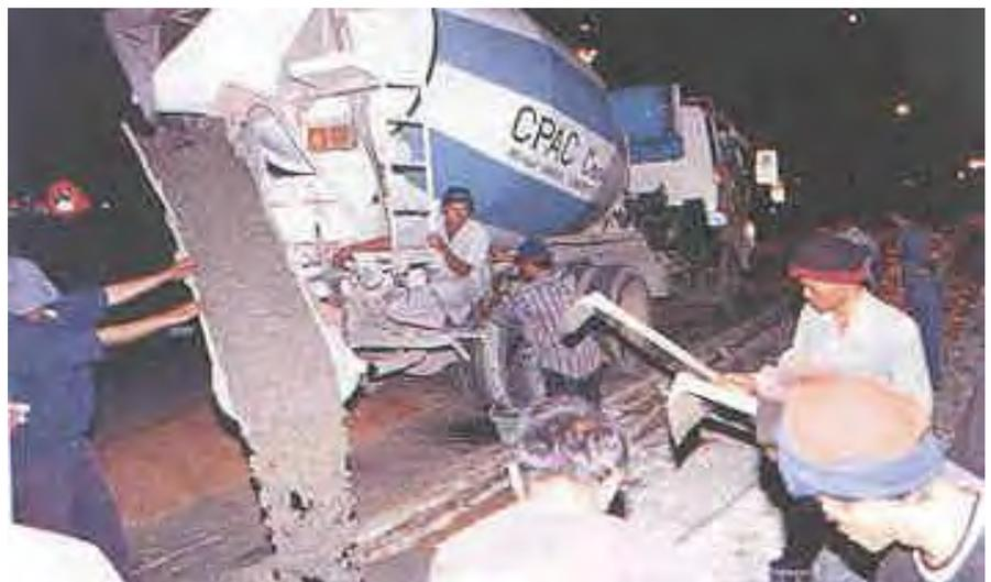
Fig. 6 Pavement Repair with High Early Strength Concrete
